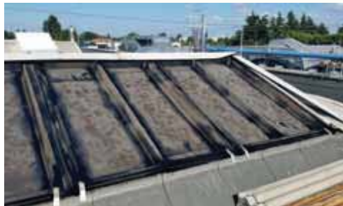
POSA BARRIERA VAPORE POLYVAP RADONSHIELD
